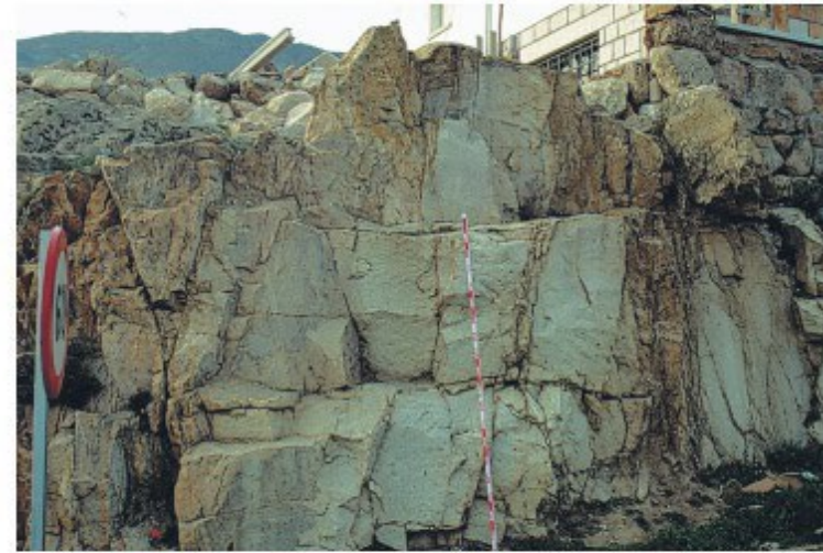
Granite. Good quality. Several sets of weathered discontinuities.
